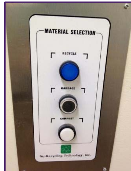
Figure 20. Button controls in chute room
