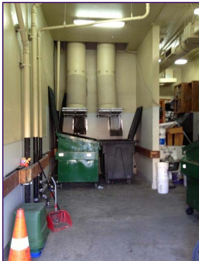
Figure 18. Trash room with dual chutes
