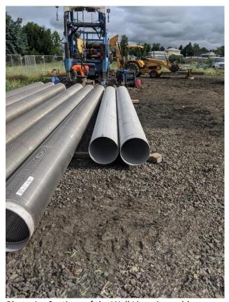
Photo 1 – Sections of the Well Liner Assembly
