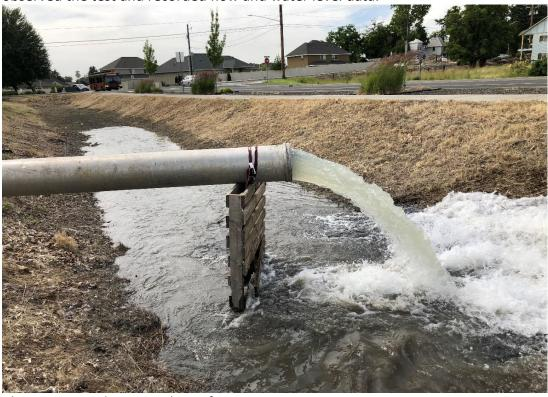
Photo 4 – Groundwater Discharge for Pre-Step Test.
