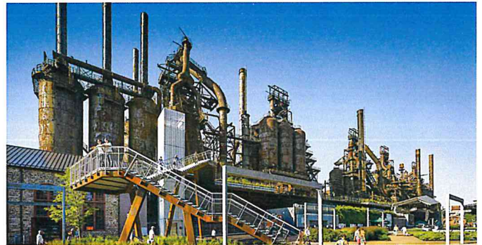
HOOVER-MASON TRESTLE | Bethlehem, PA
