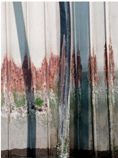
Dock piling damaged during high seas event.
