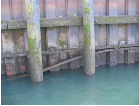
Deteriorating condition of the sheet pile wall housing the high dock, December 2021
