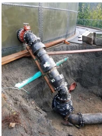
2018 Reservoir Seismic Valve Installation
