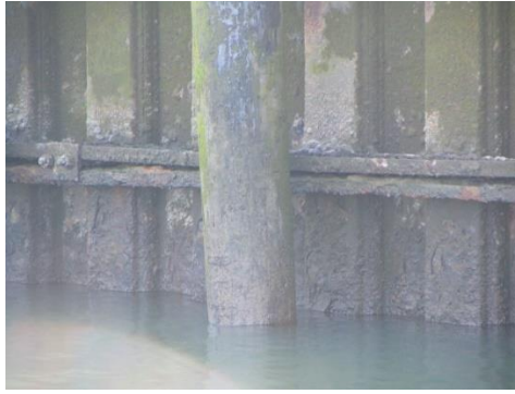
Deteriorating condition of the sheet pile wall housing the high dock, December 2021
