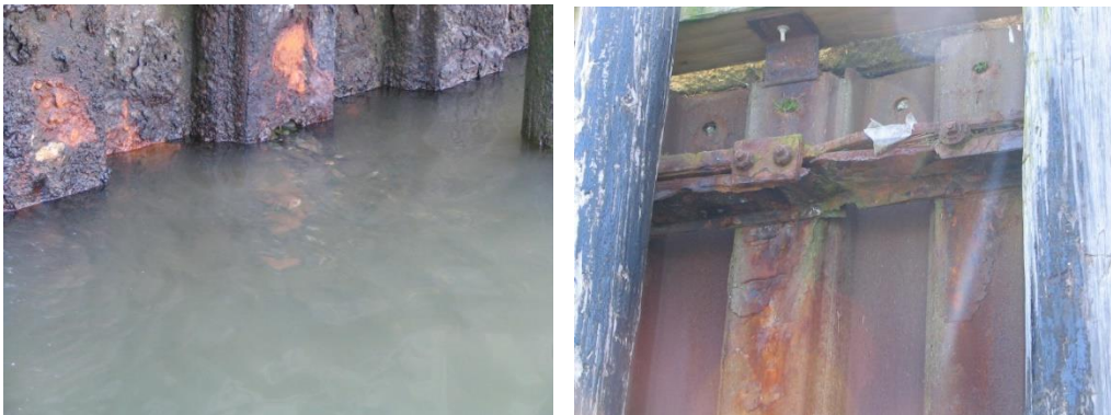
Deteriorating condition of the sheet pile wall housing the high dock, December 2021
