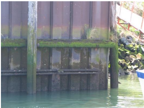
Deteriorating condition of the sheet pile wall housing the high dock, December 2021
