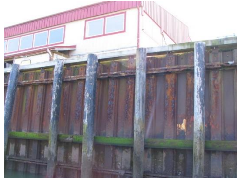
Deteriorating condition of the sheet pile wall housing the high dock, December 2021
