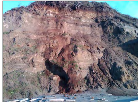
Image 1 Coastal erosion Nesika Beach
