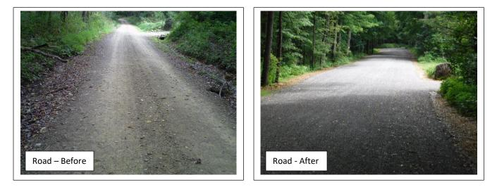
**Problem:** The road was severely entrenched, with severely eroded ditches. The deep ditches were carrying sediment to the stream. The entire roadway had flooding and erosion problems.
