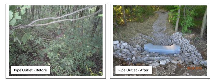
**Problem:** A large amount of stormwater was concentrating between two Township roads, causing a severely eroded gully to form. Existing crosspipes were too small. The outlets of the existing crosspipes were failing, causing the surrounding banks to erode.
