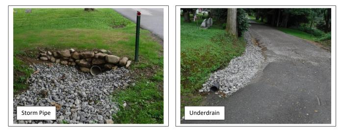
**Problem:** Water from a paved parking area was running onto the Borough road, causing erosion and carrying sediment directly to the river. Water was laying in the existing ditches since there were no outlets. The existing road profile was lower than the surrounding area.
