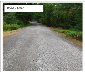
**Problem:** The existing road was entrenched and had inadequate drainage, causing the base to become unstable. Existing, deep ditches were discharge directly to nearby stream.
