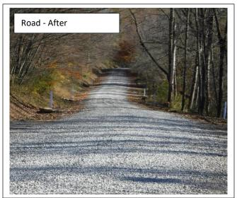
**Problem:** Existing cross pipes were undersized, and there were not enough. Severe erosion was occurring at the outlets of the existing cross pipes. The poor drainage was causing the road base to become unstable.
