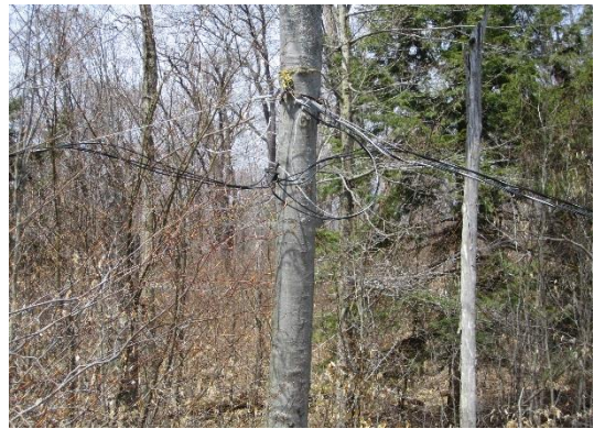
Figure 9 Power line in trees
