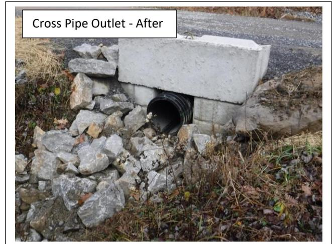
**Problem:** The existing cross pipes were too small, causing erosion at the outlet of the pipes. Standing water in some of the roadside ditches was causing water to saturate the road base, creating potholes. The lack of head and end walls on the existing cross pipe was causing the road bank to erode.
