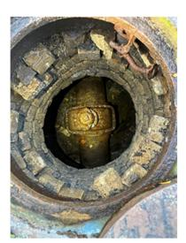
the Calendar Year 2024 budget for the replacement of these six non-operable water shut-off valves. Replacement will include new valve vault structures to upgrade from existing brick and mortar structures for safety and stability as well as installing new butterfly valves to replace the failed gate valves.
