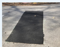
Permanent asphalt patching in the road.
