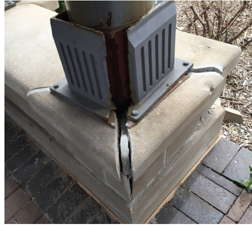
Examples of water damage
