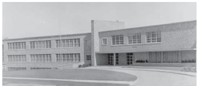
(Edgewood Middle School ca. 1959 Photo credit: Highland Park Historical Society)
