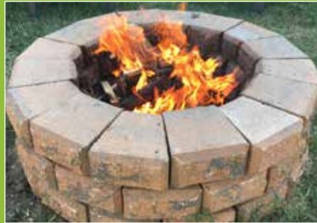
Permanent fire pit structures require a building permit.
