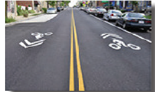
Typical Shared Roadway Pavement markings – the “sharrow”
