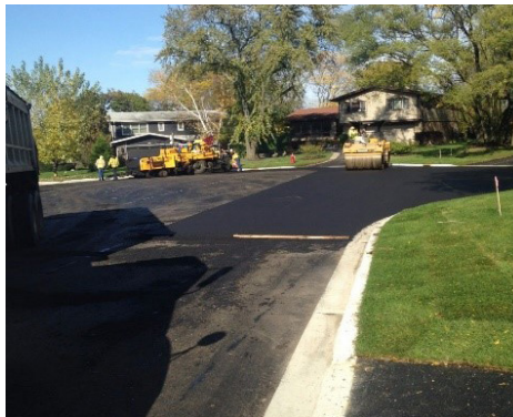
The Charal Ln. Watermain Replacement Project improved water circulation in a closed pressurized watermain distribution system, improved the storm sewer, and replaced the old concrete pavement with new asphalt.
