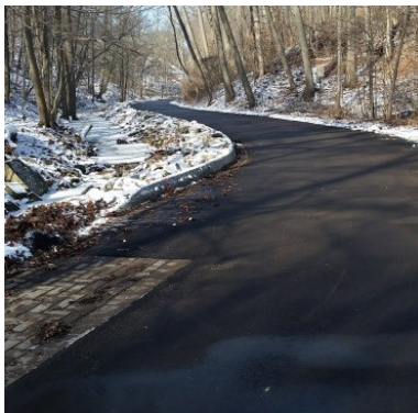
The Ravine Dr. and Hawthorne Ln. watermain and roadway reconstruction project entailed upsizing of an aged watermain, installation of new curbs, and reconstruction of roadway.
