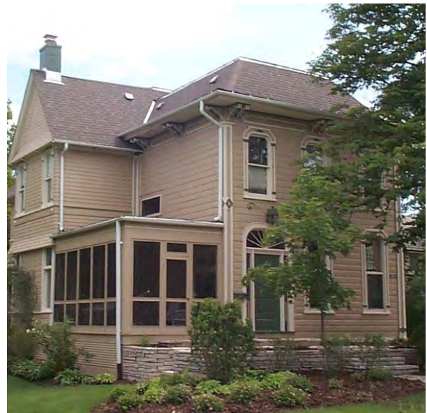
Figure 1: 120 Belle Avenue, one of the first local landmarks
