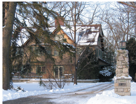
"Thornecote" c.1901 215 Prospect • Howard Van Doren Shaw National Register of Historic Places Landmarked: 1987
