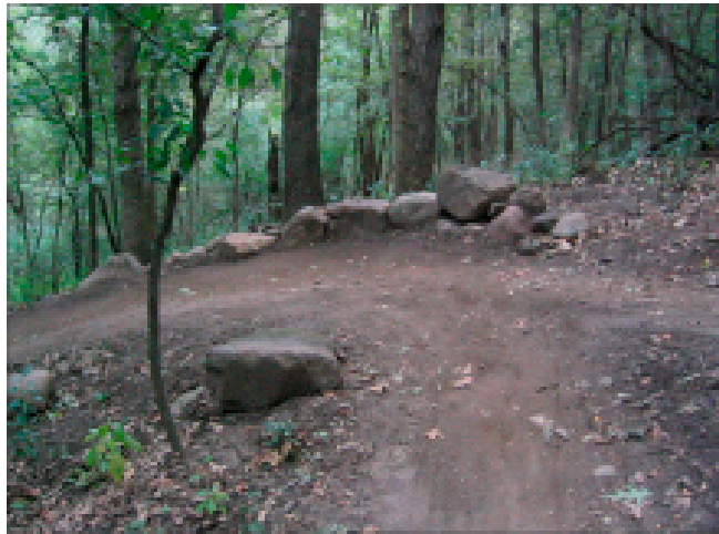
A superelevated trail curve plus embedded rocks along trail edge
