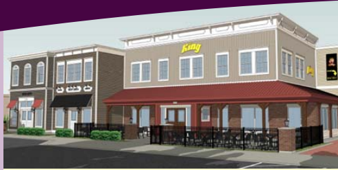
BBQ King & American Legion expansion are now under construction in Downtown Huntley
