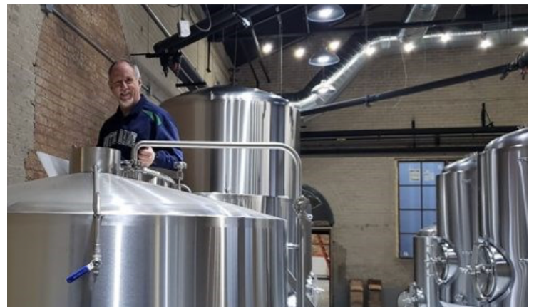
TERRY HITPAS CHECKS THE FITTINGS ON THE NEWLY INSTALLED TANKS AT SEW HOP'D BREWERY
