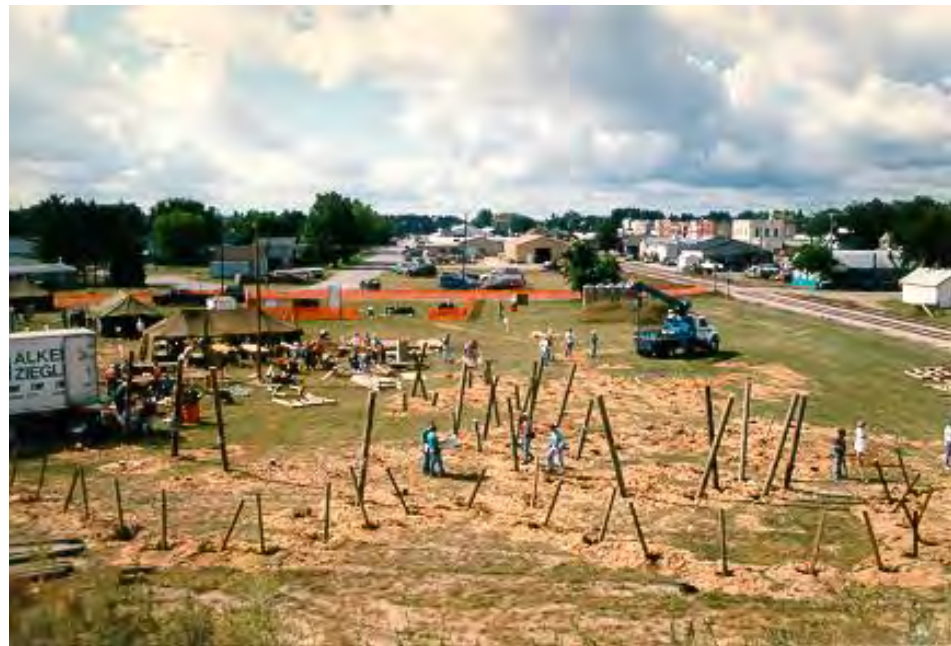
Construction, Village of Kalkaska
