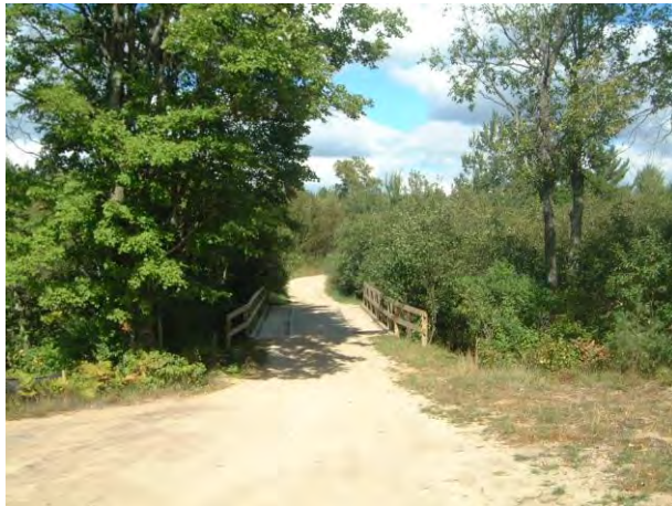
Boardman River Bridge, Boardman Township
