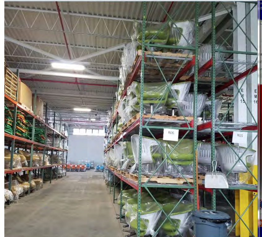
Storage too close to sprinkler system
