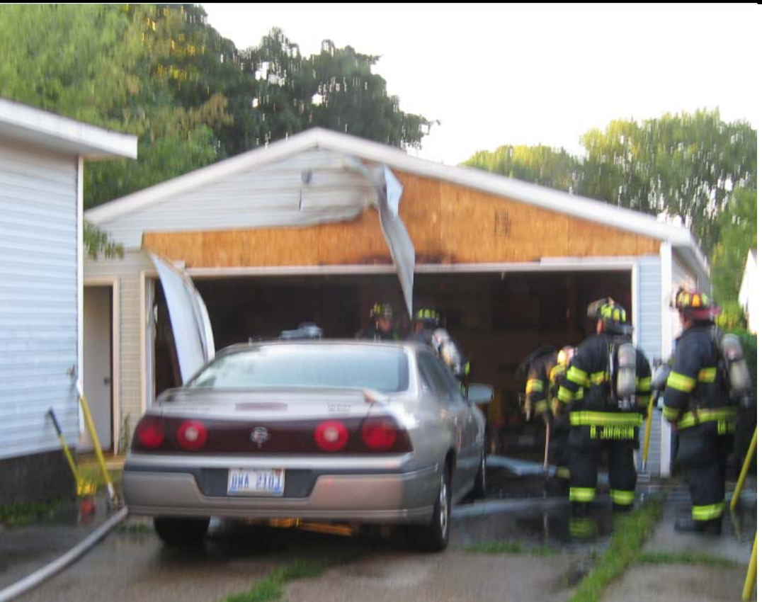
July 23, 2020 car fire on 58th St. also damaged siding on garage and house
