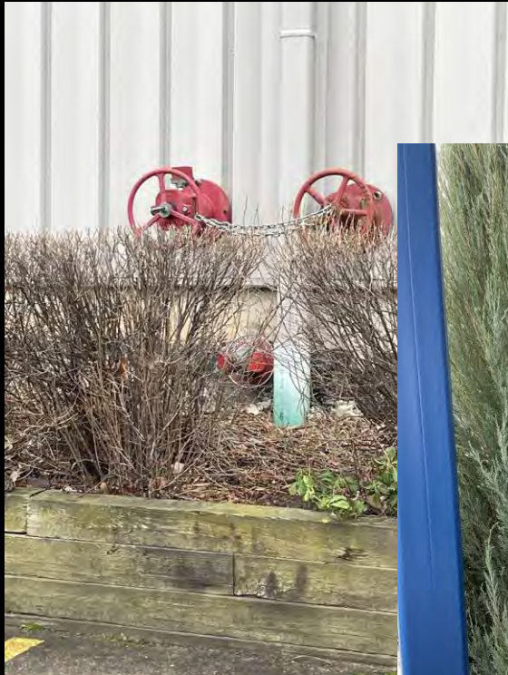
Inaccessible suppression equipment
