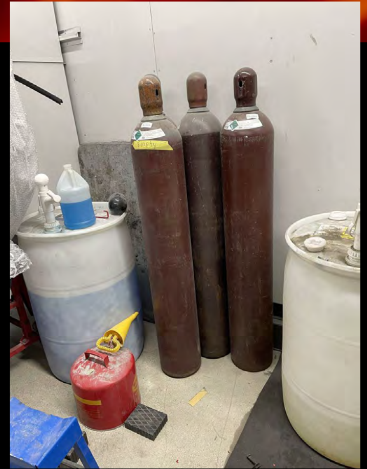
Tanks not secure; chemical containers not labeled
