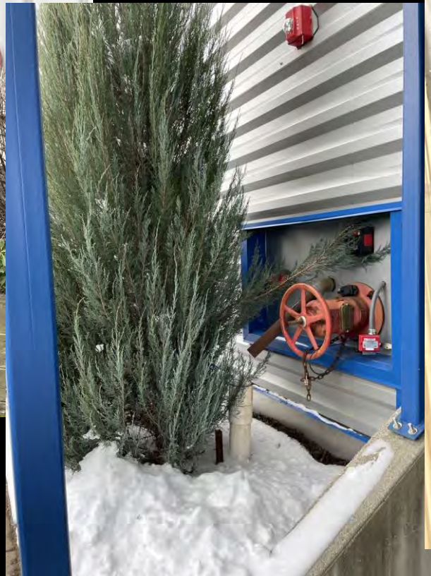
Inaccessible suppression equipment
