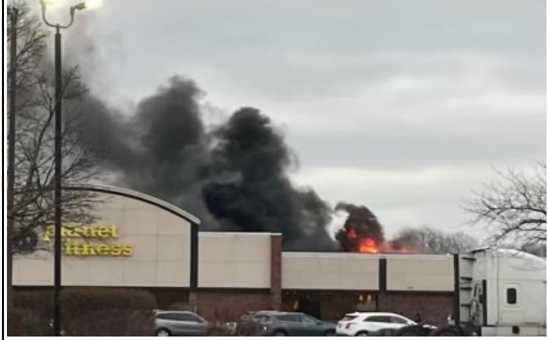
Photo from passerby at 5270 Eastern on December 11, 2021. Investigation determined that fire started in the rooftop HVAC unit and spread via high winds to the roof membrane.
