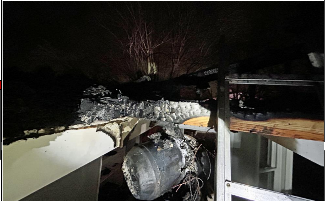
Stauffer Ave. duplex, 12/27/23; residents at home, but initially unaware of fire. Neighbors across the street called 9-1-1. Flames were coming through the roof when fire fighters arrived. Investigators determined fire originated in attic in area of can light fixture attached to bottom chord of truss.
