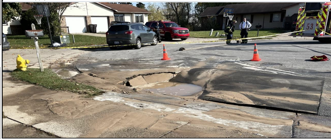
Watermain break near hydrant required change in water supply.
