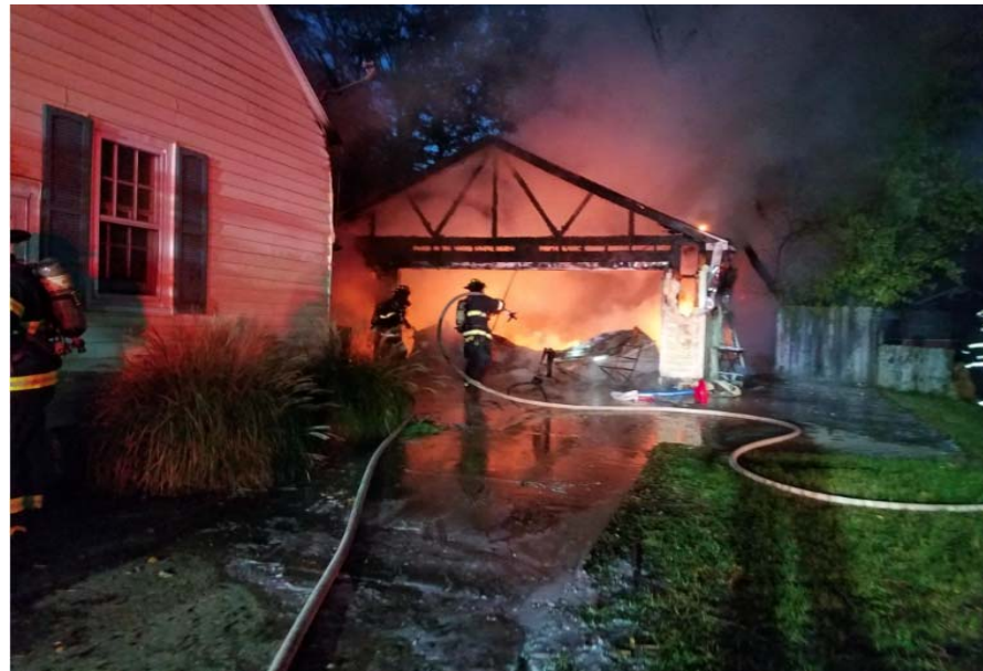
Garage was destroyed and there was some damage to the house. Cause remains unknown.
