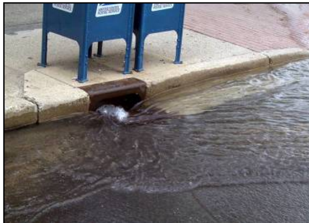
Storm water runoff entering the storm sewer after a rainstorm.
