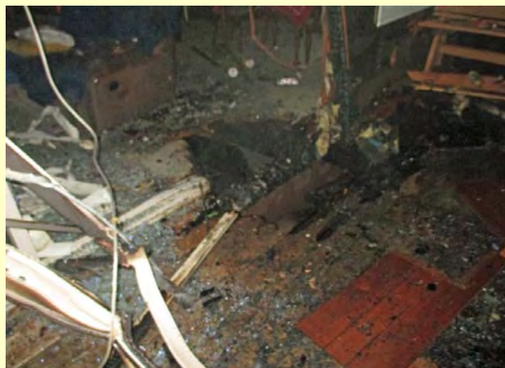
February 6 – 4679 Kimball – fireplace ashes placed on deck burned through the threshold of the slider and into the interior of the home.
