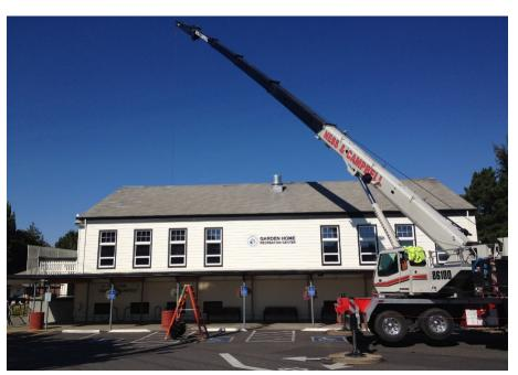
Scope of work included a 36'x36' steel play structure, bracing for the existing fire suppression piping, steel brackets and bracing for existing boilers, seismic bracing to support brick chimney structure, Simpson hardware and sheathing at entrances and skybridge connections, structural concrete foundation and steel moment frame to support skybridge, seismic expansion joints, ledger bracing in gymnasium, asbestos abatement,
