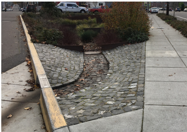
Street-side Low Impact Development (LIDA) swales
