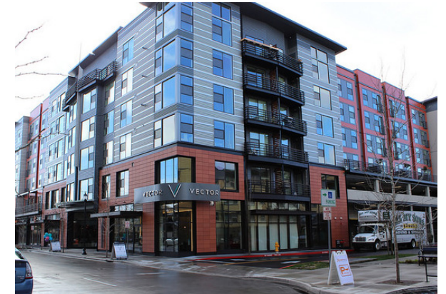
Example from Orenco Station of 4-5-story mixed use building with retail on the ground floor and residential units above.
