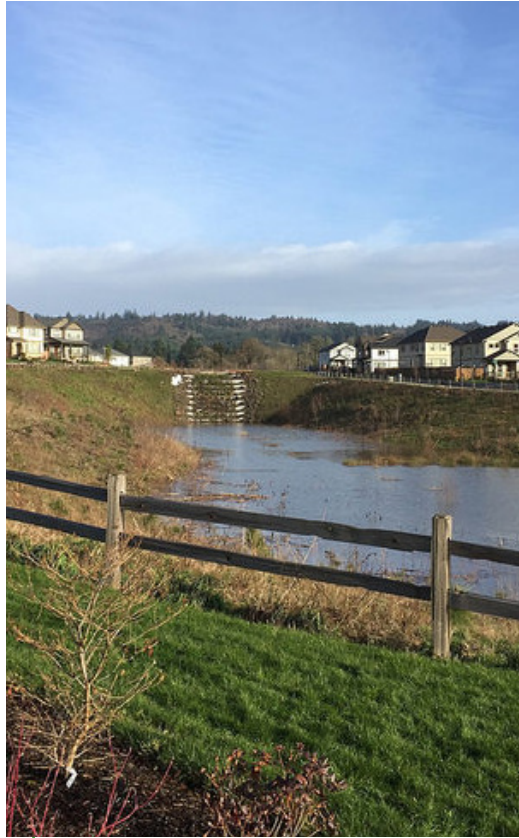
Active stormwater management pond surrounded by park and walking trails
