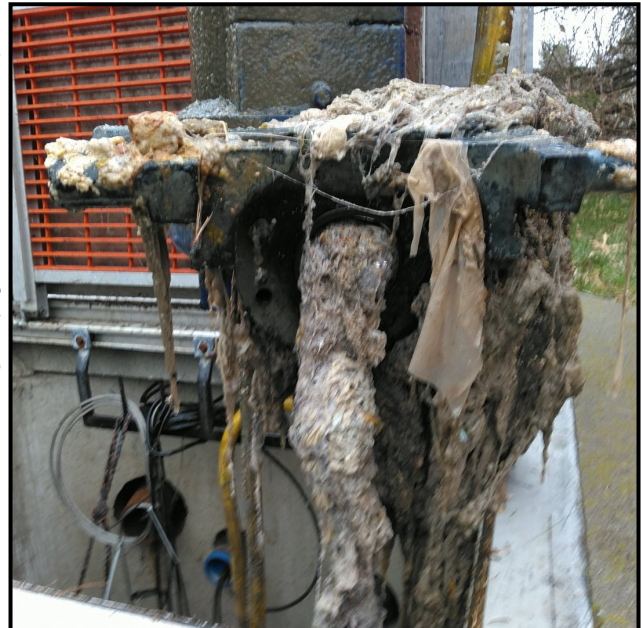
Pump recently pulled at a Village lift station due to residents flushing items other than toilet paper.
