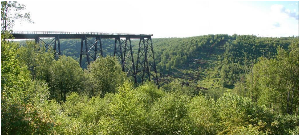
Figure 45. Kinzua Bridge following a 2003 tornado that destroyed much of the original steel viaduct. Photo credit: David E. Casteel.
