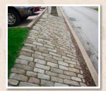
Use infiltration features for roadside drainage system
