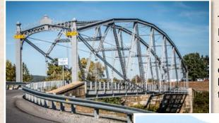
The nearly 288-foot long Pine Creek Lenticular Truss Bridge near Jersey Shore is one of only about 50 truss bridges still standing in the United States.
