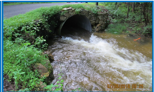
Above: Penn Township, Beetem Hollow Road: next stream culvert to be replaced with a 14 ft box culvert. Note the back water scour to the left of the inlet pipe. Construction is anticipated for Summer 2019.
