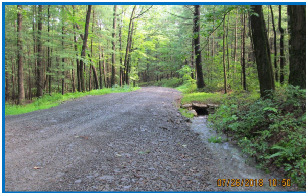
Above: Dickinson Township, Cold Springs Road: Base Material placed Spring 2018 to create a crown (center slope on the road profile) showing a shallow cross pipe that was replaced in 2016.
