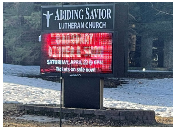
Example: non-masonry base, with masonry planter around sign (non-compliant sign).
