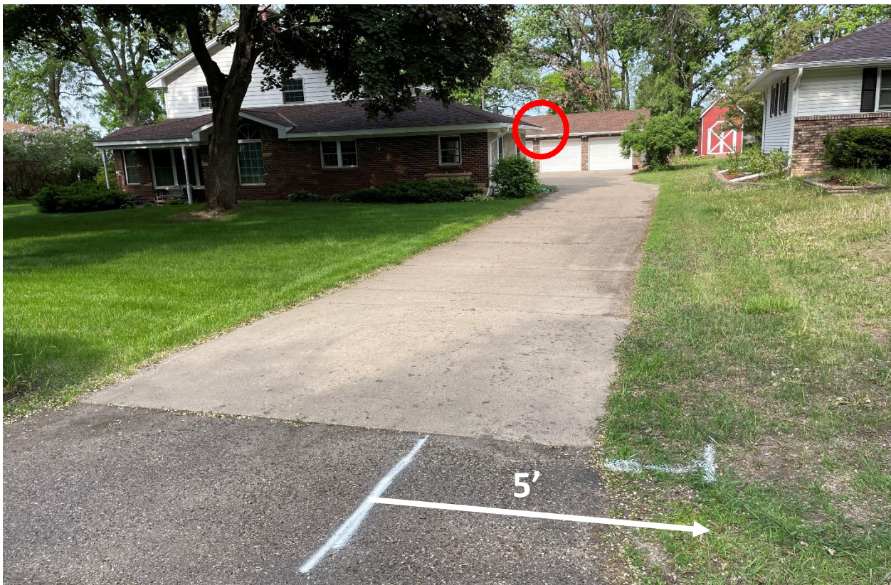
7850 Spring Lake Road (photo May 25, 2023). Non-conformity: driveway is setback less than 5' from side yard property line. Homeowner has requested a Variance to keep as-is. Homeowner plans to replace driveway. If entire driveway were to comply with 5' setback driveway would likely shift toward house, creating a pinch point where roof soffit hangs over driveway (red circle). Staff recommends keeping the driveway as-is.
