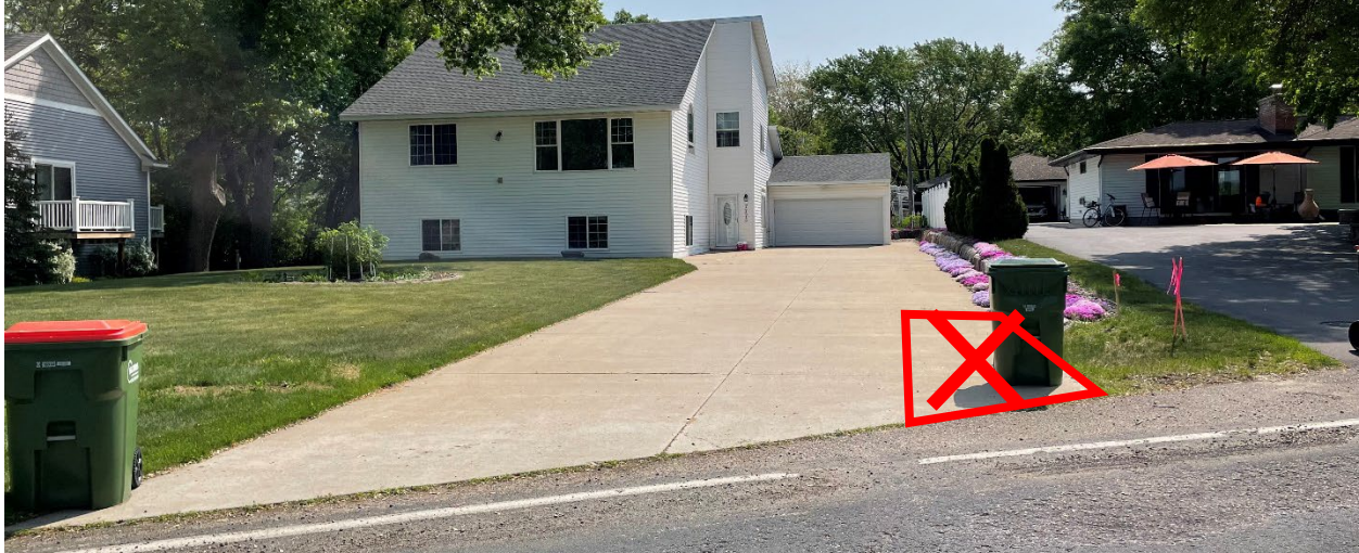
7775 Spring Lake Road (photo May 25, 2023). Non-conformity: south (right) setback is less than 5' (0'). Staff recommends installing the apron with a 5' side yard setback. Homeowner has requested a Variance to keep as-is. Resident has special needs. A bus accesses the driveway frequently for pick-up/drop-off.
