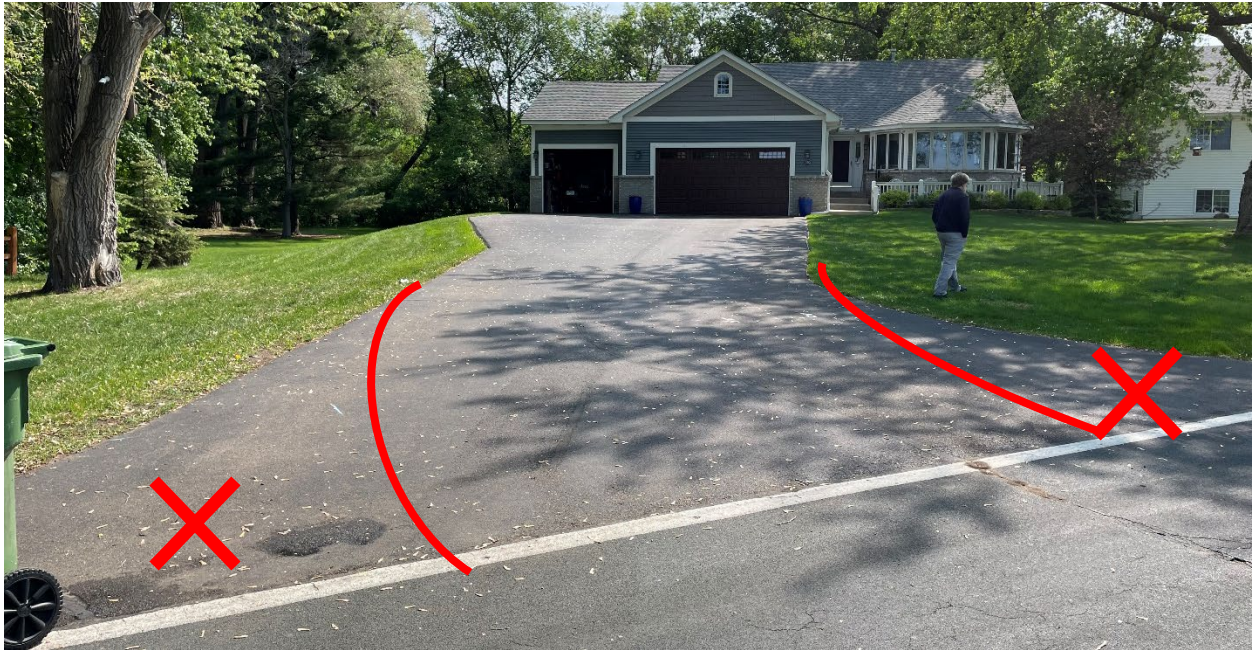
7785 Spring Lake Road (photo May 25, 2023). Non-conformity: driveway exceeds 24' width (41') at street. Driveway is 24' at property line. Homeowner has requested a Variance to keep as-is, or as close to as-is as practical. Driveway is on a curve. A wider driveway would be easier to enter from southbound traffic.
