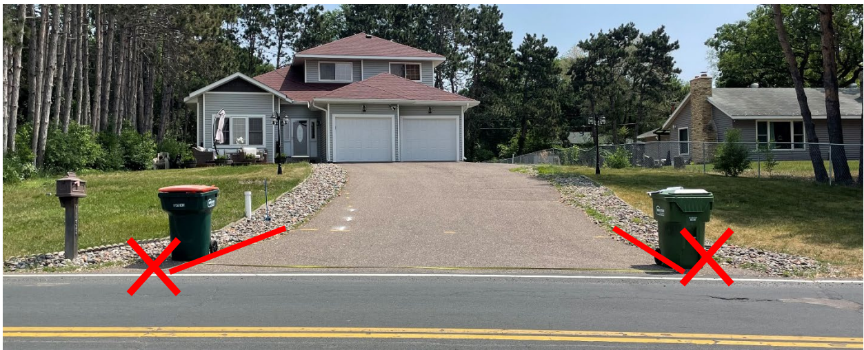
7735 Spring Lake Road (photo June 8, 2023). Non-conformity: driveway is wider than 24' at ROW. Staff recommends installing 24' wide apron. NOTE: Staff did not mail a non-conforming notice to homeowner, mistakenly interpreting the ROW as further from the street (ROW is about 1' or less from street). It is the driveway wings that are non-conforming.
