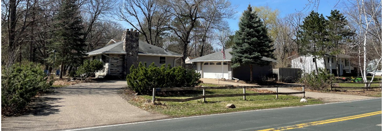
3001 County Road H2 (photo April 18, 2023). 2 nd Driveway is legal non-conforming because the City issued driveway permits in 1996, and 2003 (2 nd driveway is evident on 1974 aerial photo, and possibly established at the time of home construction in 1950's).
