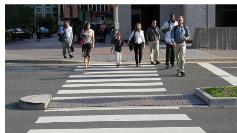
Pedestrian safety island with raised concrete "nose" and paver median
