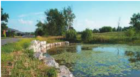
Shoreline enhancements around the perimeter of detention ponds
