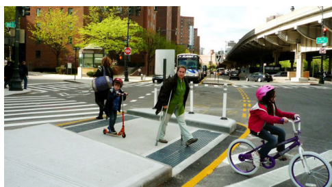
Pedestrian safety island with raised concrete "nose" with warning bollards and plates
