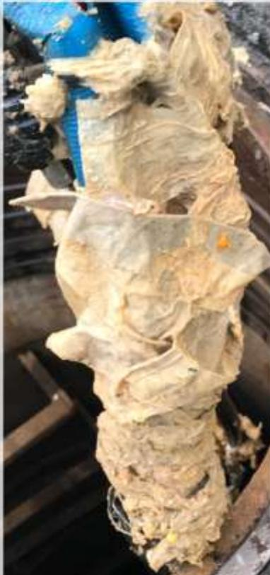
Flushable wipes have cost the City in excess of \$25,000. On March 19<sup>th</sup> the Groveland Lift Station became clogged with flushable wipes, causing a costly repair due to the damaged grinder and motor.
