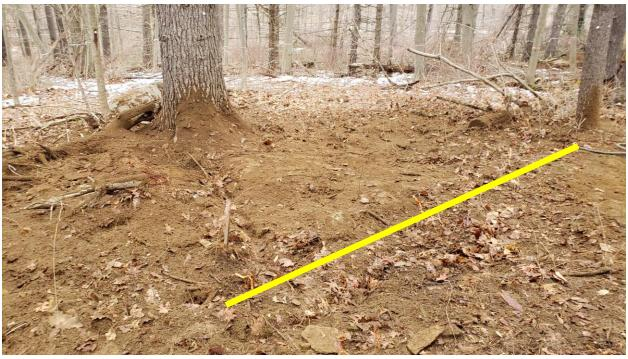
Photo showing the marked limits of where excavation can occur (yellow line). If excavation or grade change is needed between the tree and this line, the tree should be removed.
