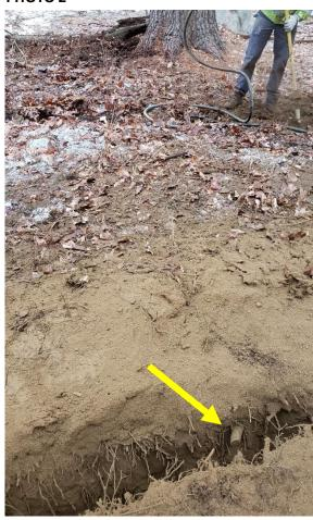
Photos 1 and 2 were taken March 17, 2023 and show the first trench that was excavated with the air spade approximately 16 feet from the base of Tree 135. There was only one root larger than 1-inch in diameter (indicated by yellow arrow). This root was pruned.
