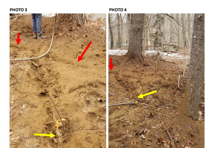
Photos showing the excavated trench at six feet from the base of the tree (red arrow) and tracing of the large root to where it was safely pruned (yellow arrow; stick with orange flagging).
