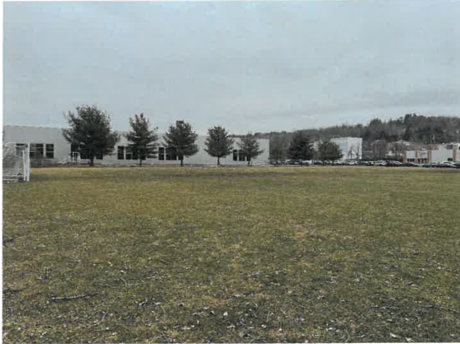
Photo No. 1 – Looking northeast from open field southcentral portion of the Site.
