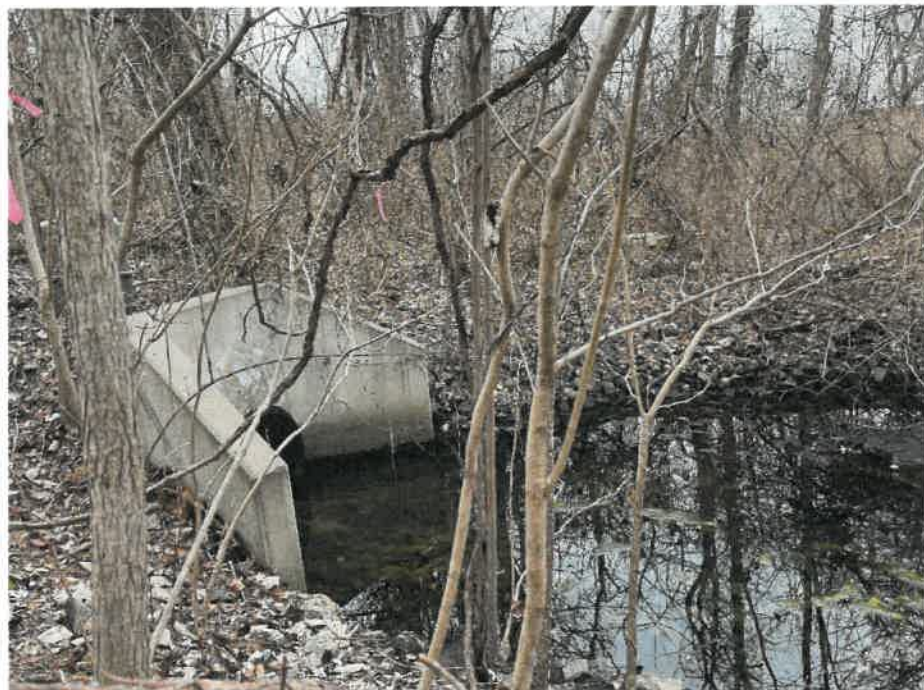
Photo No. 4 – Looking south at freshwater wetland area and culvert from the western portion of the Site.
