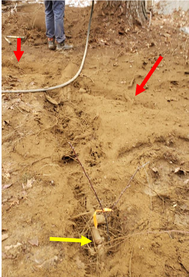
Photos showing the excavated trench at six feet from the base of the tree (red arrow) and tracing of the large root to where it was safely pruned (yellow arrow; stick with orange flagging).
