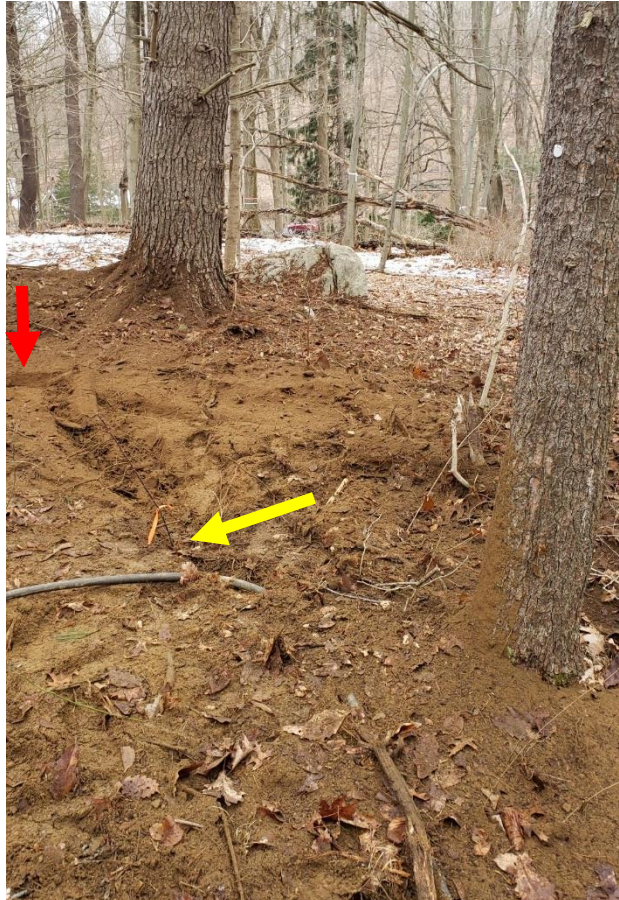
Photos showing the excavated trench at six feet from the base of the tree (red arrow) and tracing of the large root to where it was safely pruned (yellow arrow; stick with orange flagging).
