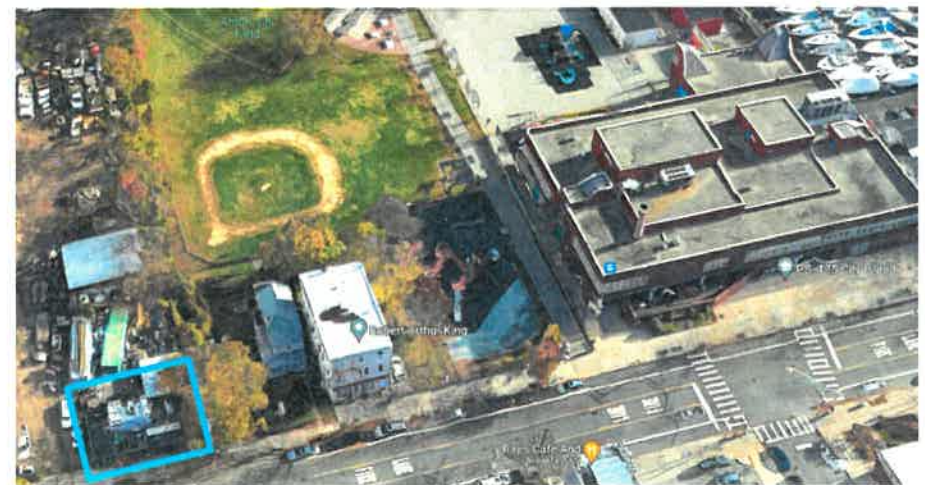
REV Demonstration Facility
