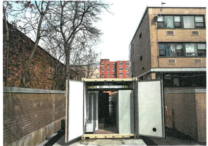
Brooklyn Facility (5+ years of operation)
