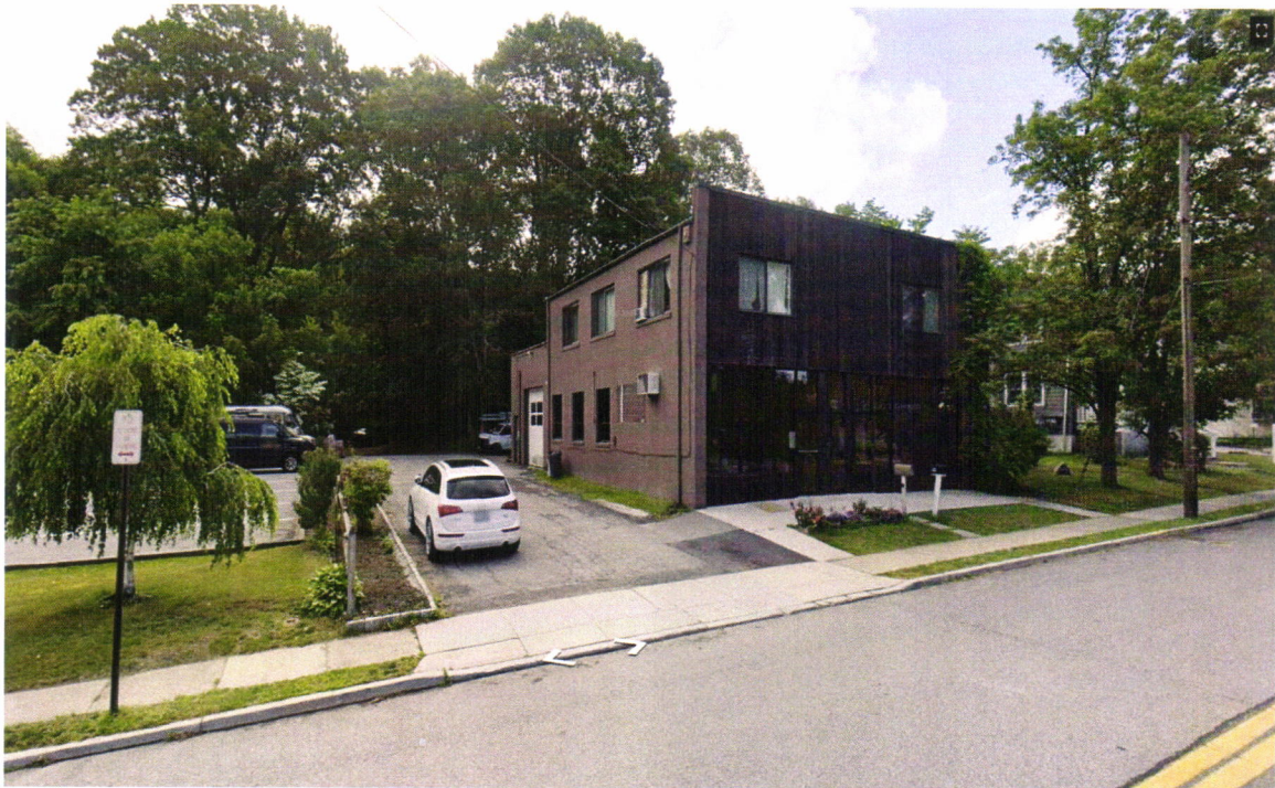
FRONT AND LEFT SIDE VIEW OF SUBJECT BUILDING - 487 LEXINGTON AVENUE
