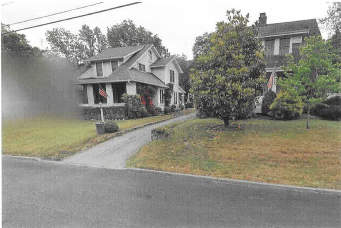
FRONT VIEW FROM BROOK STREET
