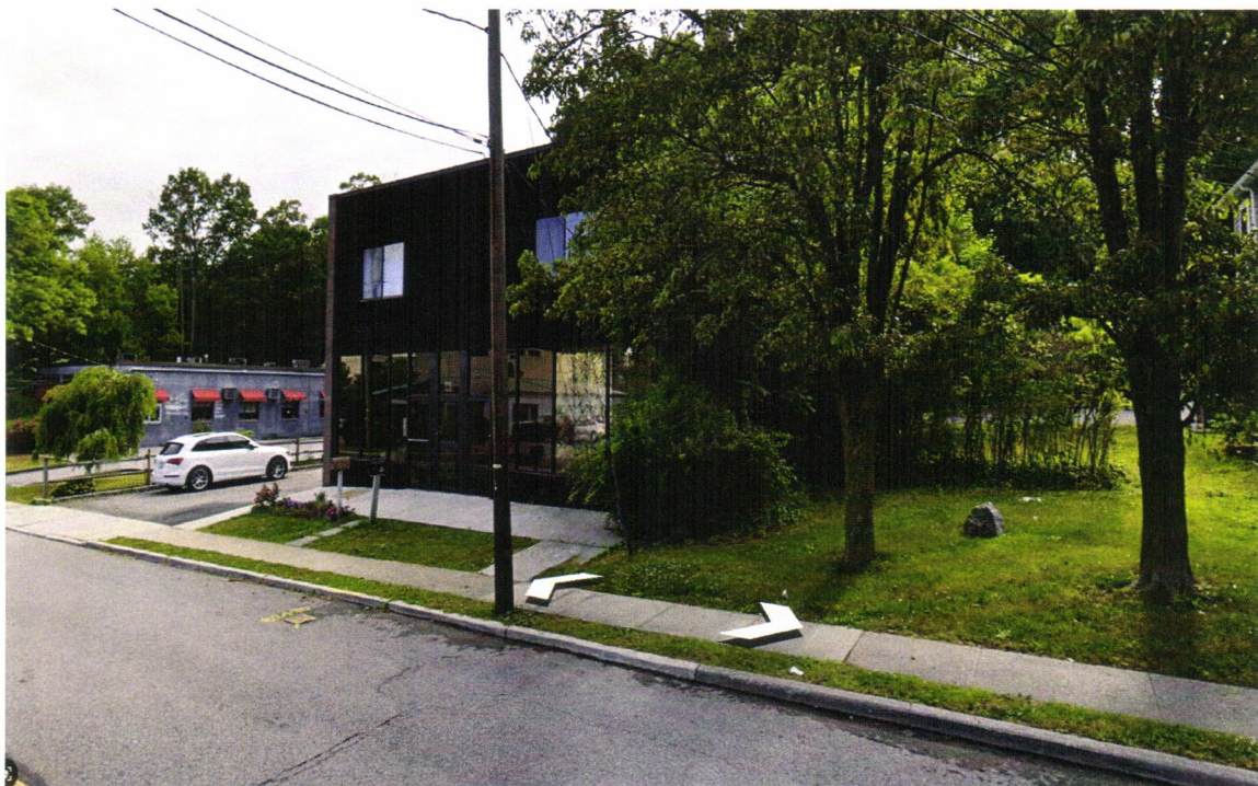
RIGHT SIDE OF SUBJECT BUILDING – 487 LEXINGTON AVENUE
