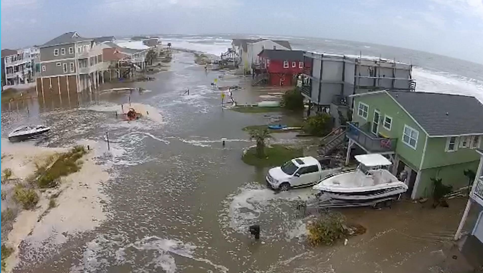
2015 OCEAN ISLE FLOODING FROM HURRICANE JOAQUIN.
