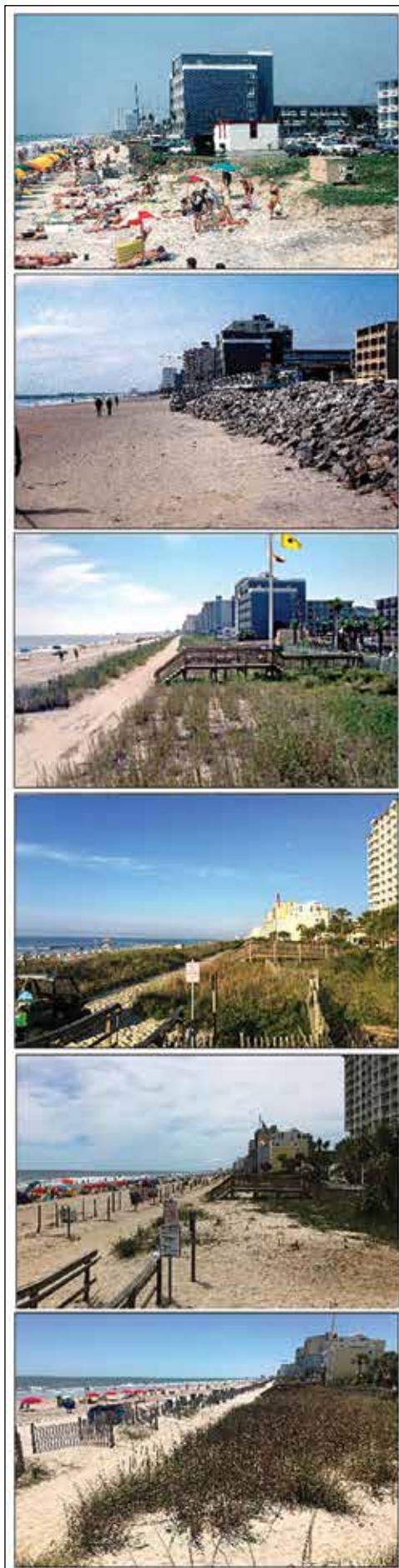
Figure 30. Myrtle Beach near 17 th Avenue South before and after nourishment. From top: Beachgoers crowded against erosional escarpments on narrow dry sand beach July 1981; wet sand beach at low tide after construction of a revetment prior to local and state bans on new seawalls — March 1985; after local nourishment by trucks in 1986, 1990, and federal nourishment by dredge in 1987-September 2001; May 2016 before Hurricane Matthew; April 2017 after Matthew; (bottom) May 2018 after vegetation recovery (photos by the authors).
