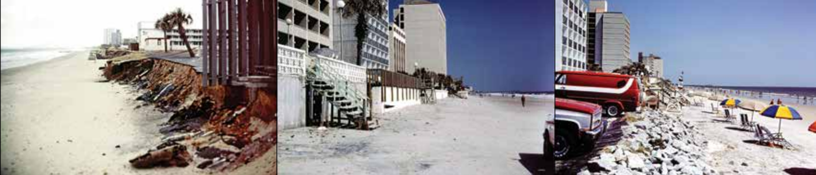
Figure 3. Eroding parking lots (1981), concrete bulkheads (1985), and riprap revetments (1985) marked the back beach before nourishment. (Photos by T. Kana.)
