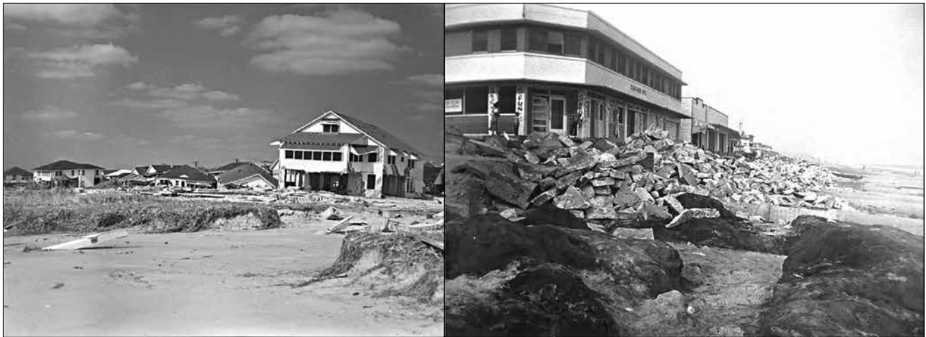
Figure 10. Post-Hurricane Hazel conditions along Myrtle Beach in October 1954. Over 80% of oceanfront structures were destroyed (left), and erosion (right) exposed underlying rock outcrops and undermined revetments. (Courtesy of Horry County, by permission.)
