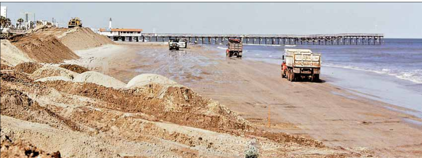
Figure 17. Interim-Phase 2 nourishment by truck from inland sources April 1986. (Source: Coastal Science & Engineering/CSE.)
