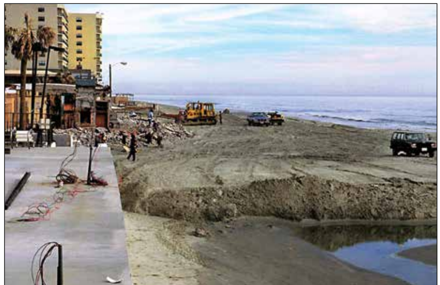
Figure 26. Post-Hugo truck-fill in winter 1990. (Photo by T.W. Kana.)
