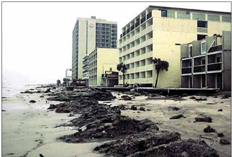
Figure 25. Hurricane Hugo storm damage at 72 nd Avenue North, including torn off roofs, undermined pools, and back beach erosion (September 1989, T.W. Kana).
