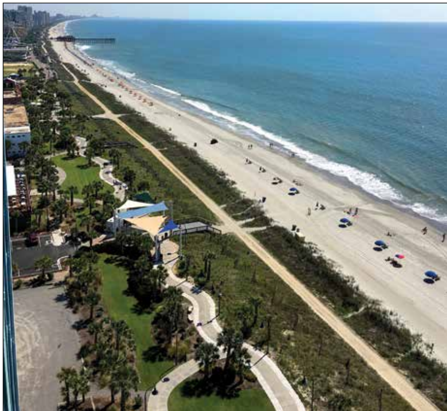
Figure 2. Myrtle Beach in 2016 showing reclaimed beachfront, which has buried seawalls and now accommodates a sinuous boardwalk, storm berm, and service road, as well as a healthy, dry sand beach. (Photo by H. Kaczowski.)
