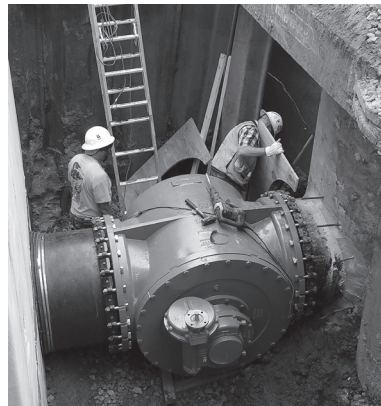
Crews install a 36-inch valve at the Fifth Avenue South sewer pump station.
