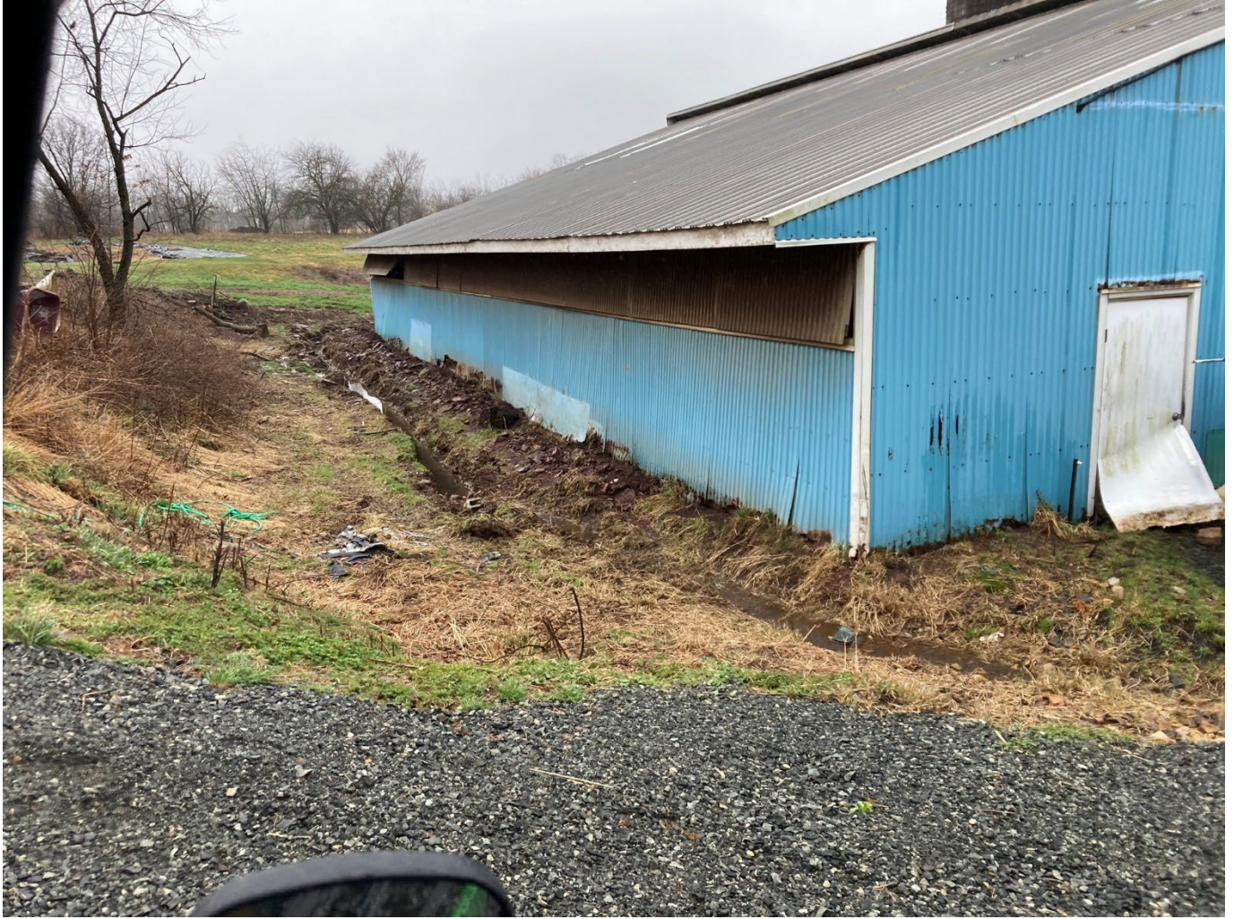
Figure 1 - Partially completed drainage improvement along existing barn.
