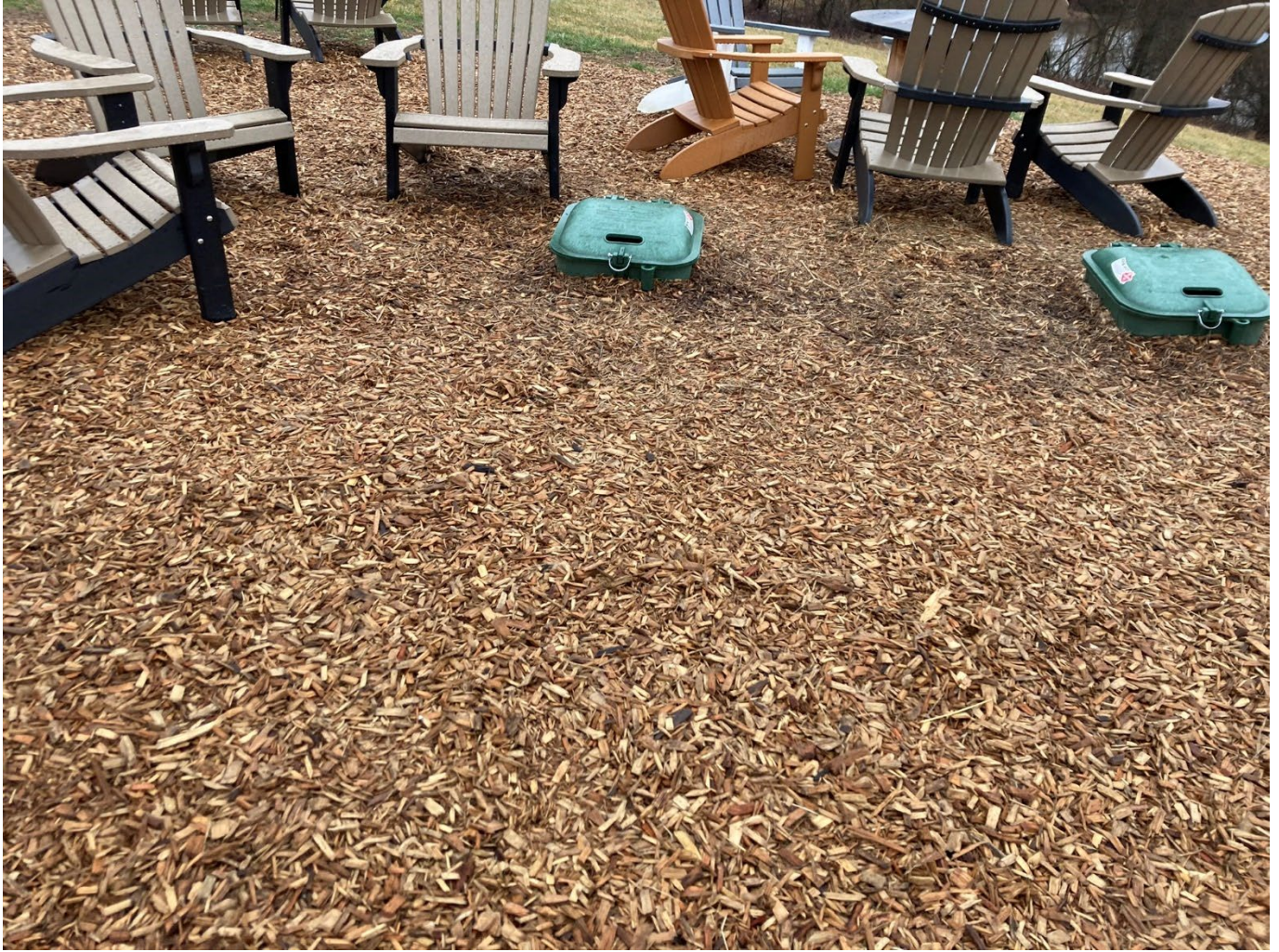
Figure 47 - View of underground propane access ports within seating area on Parcel 47-00-04324-00-3
