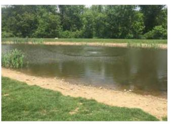
infiltration basins. The soils in these basins are specifically designed to allow for the infiltration into the soil and may contain different sized rocks, gravel, and soil. The areas are often seeded with native plants adapted to both wet and dry soil conditions. Retention basins are not the same as detention basins. Detention basins are man-made ponds designed to store water during heavy rains and drain within 48 hours.
